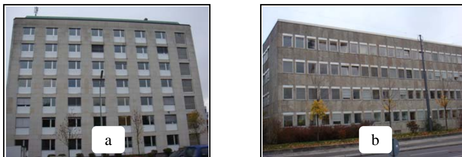
Figure 1. Facades (a and b) which seems appropriate for a good typification.
