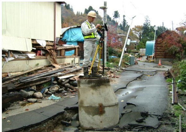
Fig.6 Surveying after the Niigata-ken Chuetsu Earthquake of 2004
