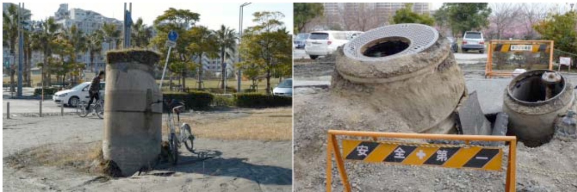
Fig. 2. Lifted manhole (left) and water storage tank (right) by soil liquefaction
