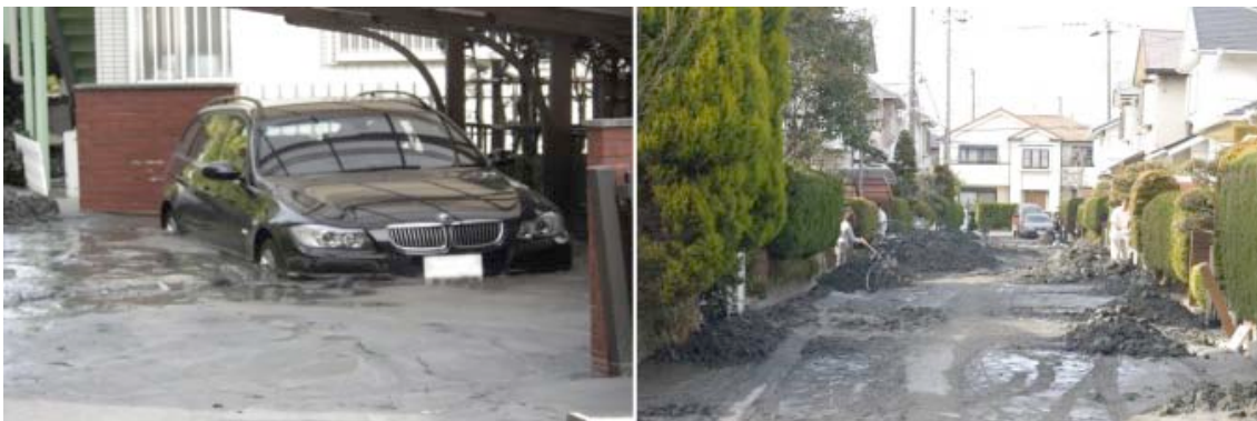
Fig. 1 Soil liquefaction in Urayasu City
